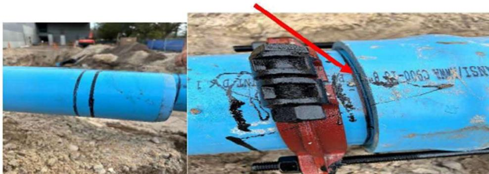
**NFPA 24-10.8.2** -The tightness of bolted joints shall be verified by the bolt torque or by the method described in the listing information or manufacturer's installation instructions.
